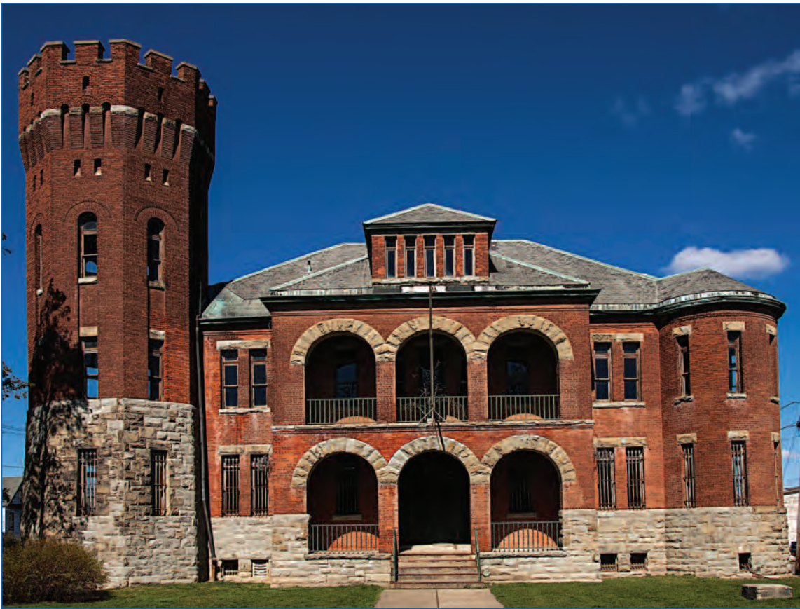
The NMTC financed the redevelopment of several downtown properties in Hudson, New York, including an historic armory that will provide space to community organizations providing educational, social, and health services programs including the Hudson Area Library and a new Senior Center. Image from CEI Capital Management.
