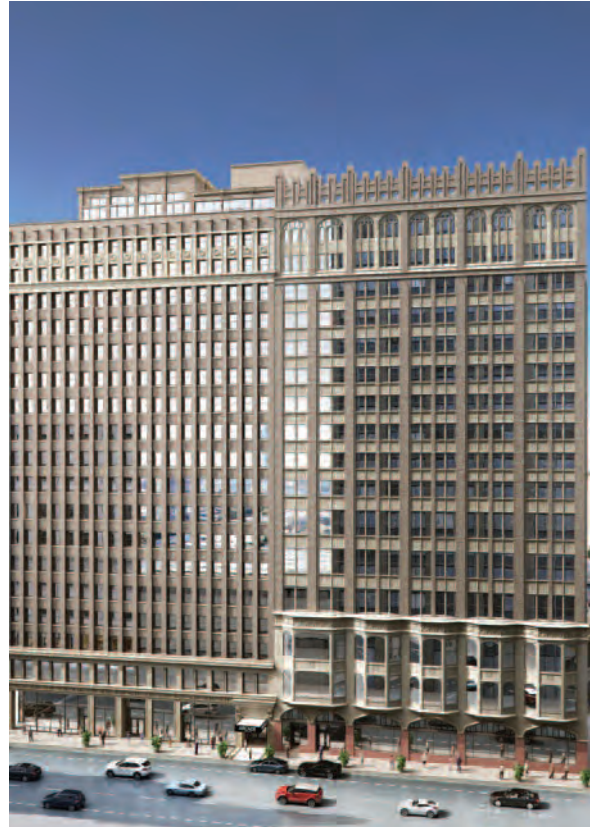
The NMTC financed the historic redevelopment of the 538,000 square foot, century year-old Arcade Building in the heart of downtown St. Louis into 282 apartments and 50,000 SF of commercial space. The building, which had been vacant for years, is slated to include 202 affordable artist lofts and 80 market-rate apartments. Image from Central Bank of Kansas City.
