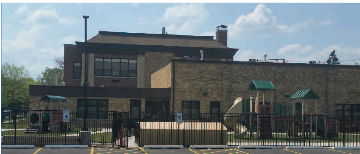
NMTC financing helped construct the Joliet Early Learning Center, a state of the art early learning program serving children 6 weeks to 12 years old from low income families in the Joliet, Illinois community. Photo by Lyle Haerle via Southside Optimal Redevelopment Advisors.
