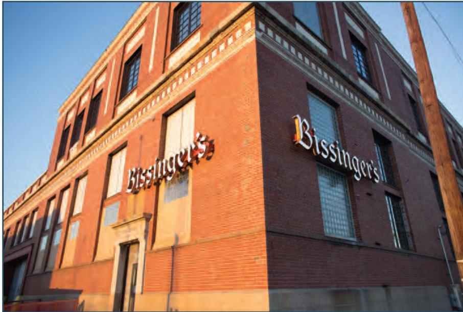
Constructed circa 1910, this historic north St. Louis building was once home to the Missouri Kansas Texas Railroad Depot. The NMTC helped finance a $15 million renovation, and the restored building will serve as the headquarters for a chocolate manufacturer. Image from Central Bank of Kansas City.
