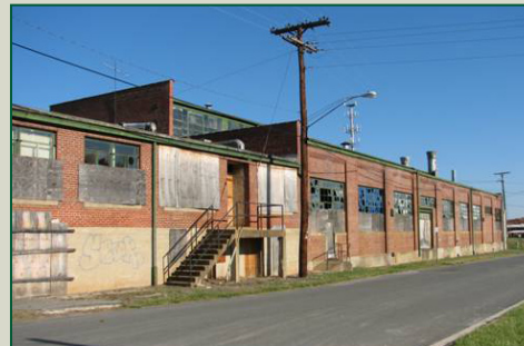
The Allen-Morrison site in Lynchburg, Virginia.
