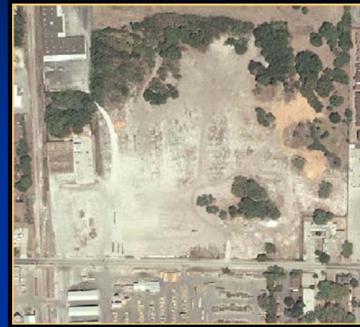
Former Robbins Manufacturing Facility
