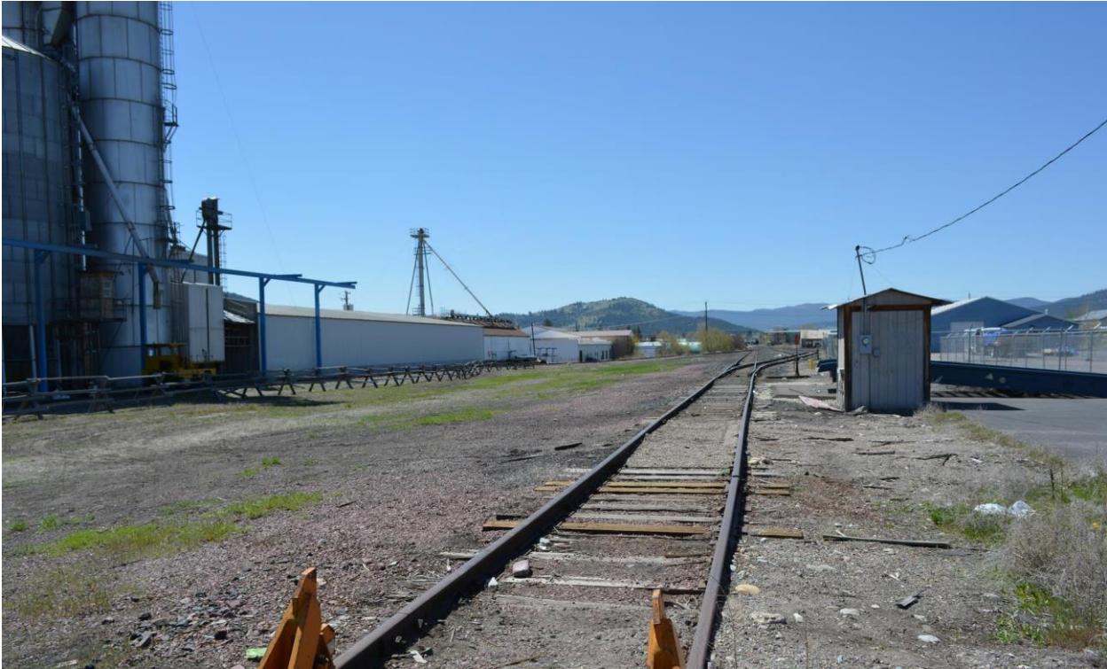
Figure 1: View behind Cenex Harvest States grain elevators
