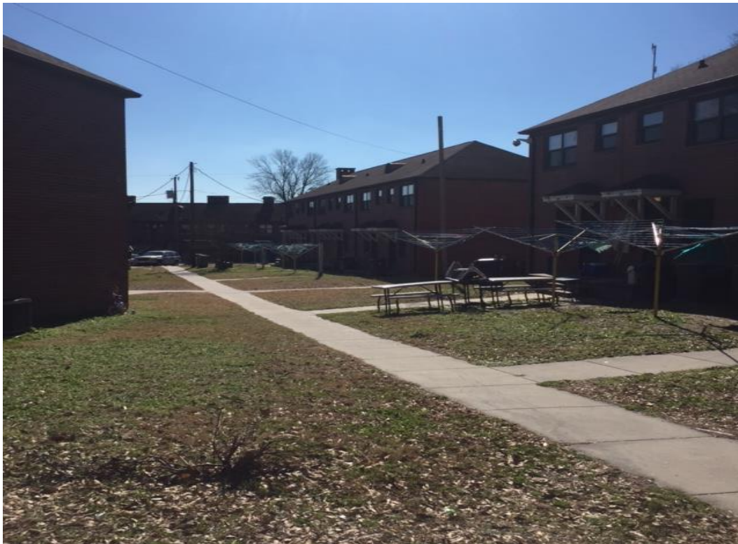
Figure 1: Trent Court Residential Buildings
