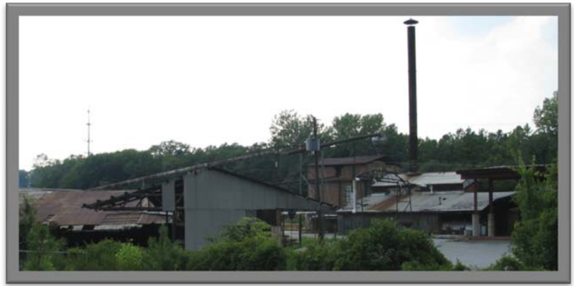
Narjoe Timber and Supply Co., just north of Atlantic Station (2010)
