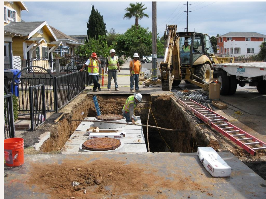
AT&T Vault Installation
