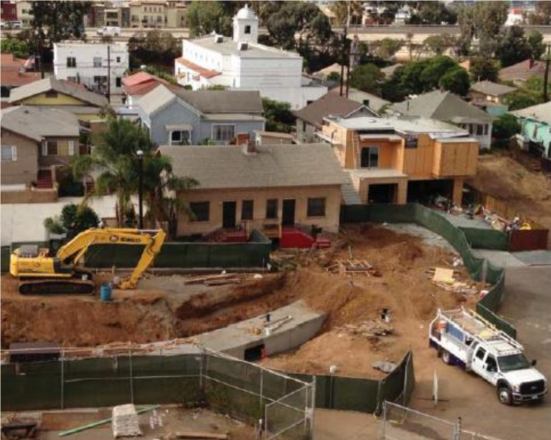
Installation of New 8' x 4' Storm Drain Box Culvert
