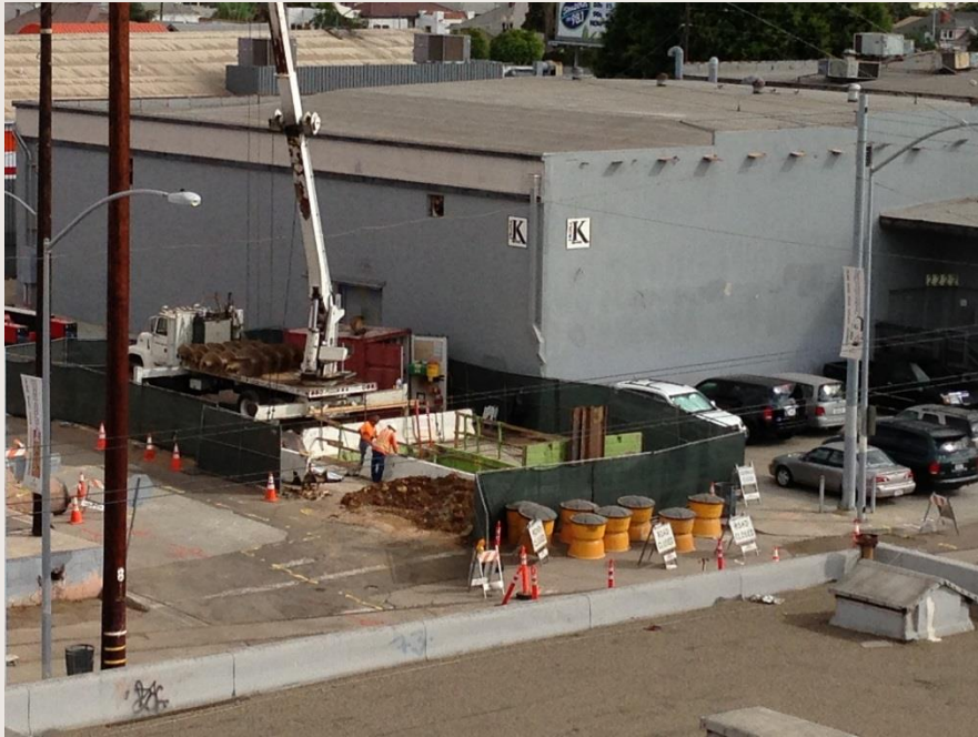
Jack and Bore of 69kV Transmission Line Under MTS Trolley Tracks
