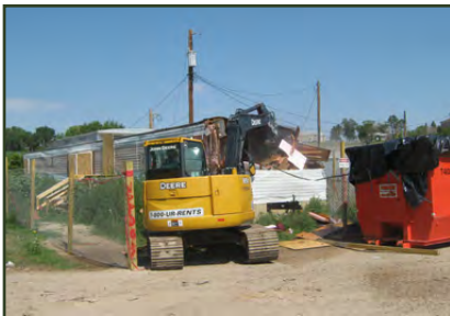
Cleanup of an abandoned house
