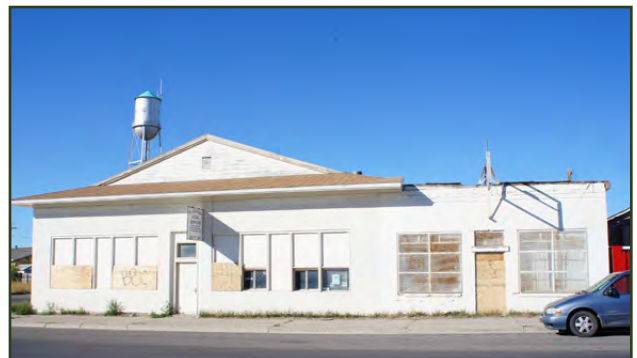
Blackfeet Mainstream building is one of 12 designated brownfield properties on the Blackfeet Reservation
