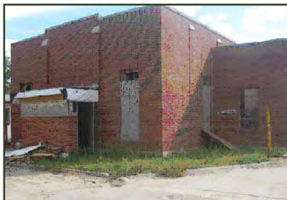
CHR Building prior to cleanup
