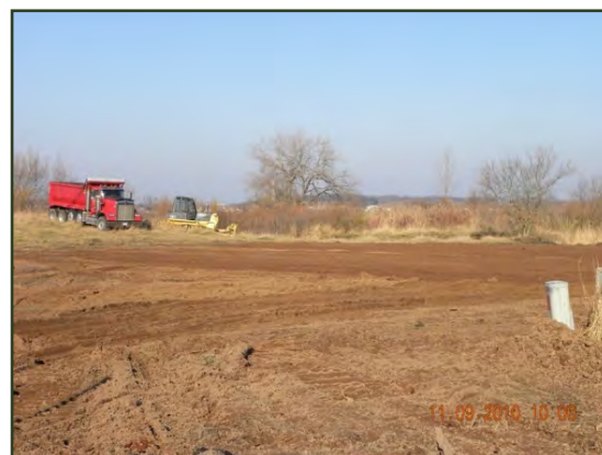
Excavation activities at the Eastlake property
