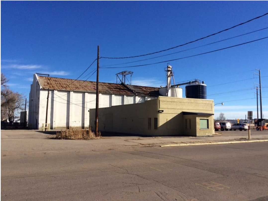
Figure 2: Former laboratory building at the Granary.
