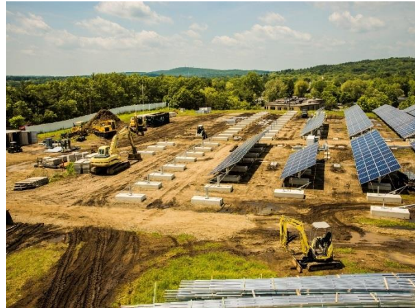
Ballast Installation
