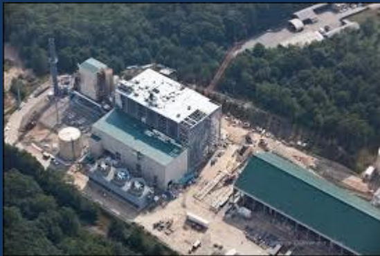
Plainfield Renewable Energy biomass power plant On former Gallup's Quarry Superfund Site, Plainfield
